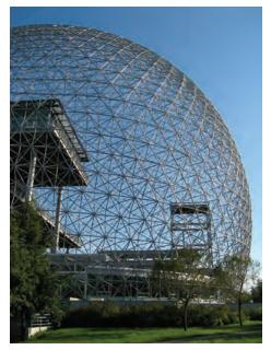
In architecture, a **space frame** is a truss-like, lightweight, rigid structure that makes a geometric pattern. Space frames can span large areas. They are strong because of the pattern of repeating triangles.
